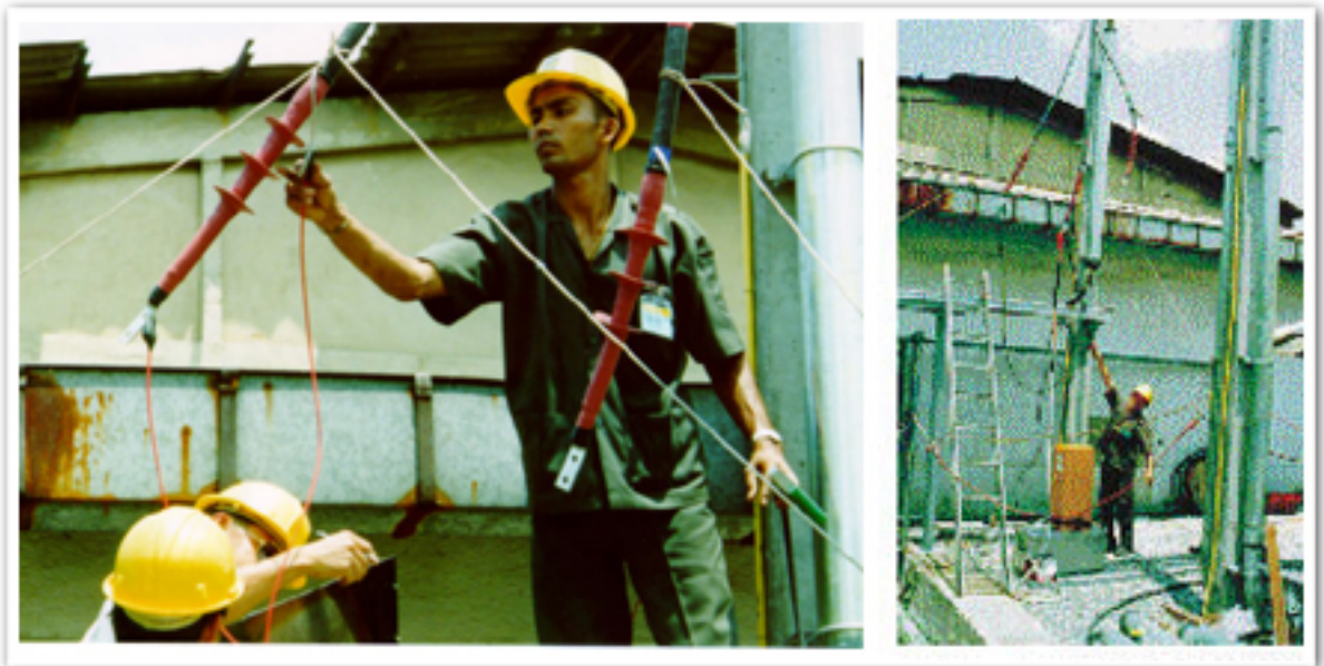
"Raychem" Field Termination Kit Installation
