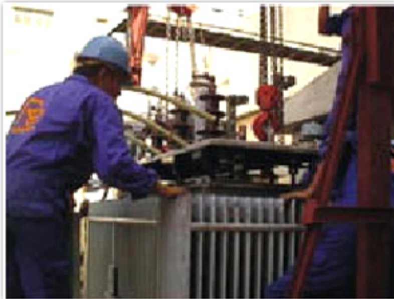
Distribution Transformer Untanking & Overhauling
