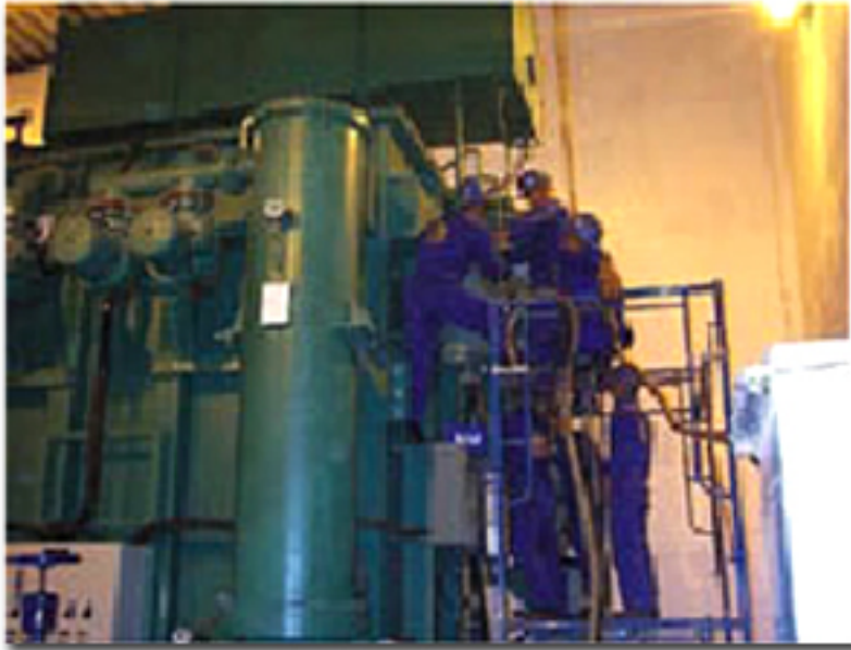
On Site Power Transformer Overhauling
