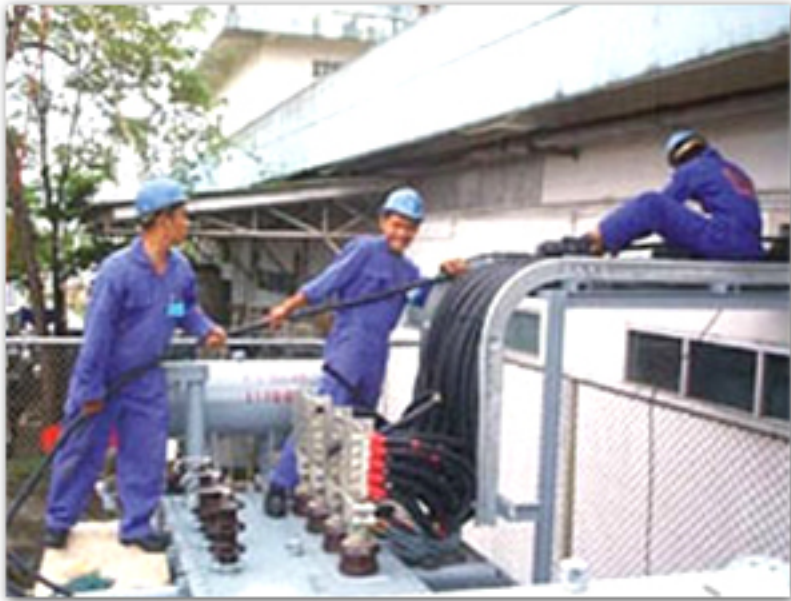
New Transformer and Low Voltage System Installation
