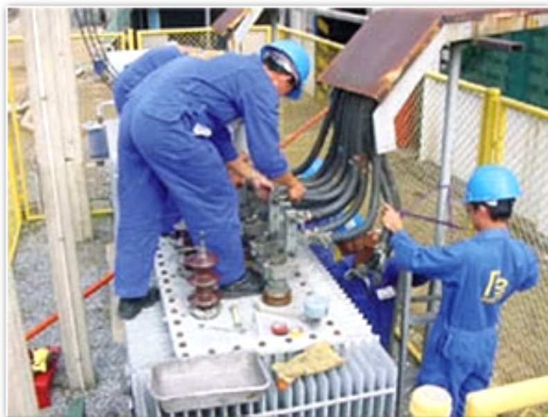
2000 KVA. 22 KV Distribution Transformer Preventive Maintenance
