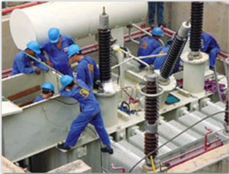
25 MVA. 115 KV. Power Tranformer Preventive Maintenance
